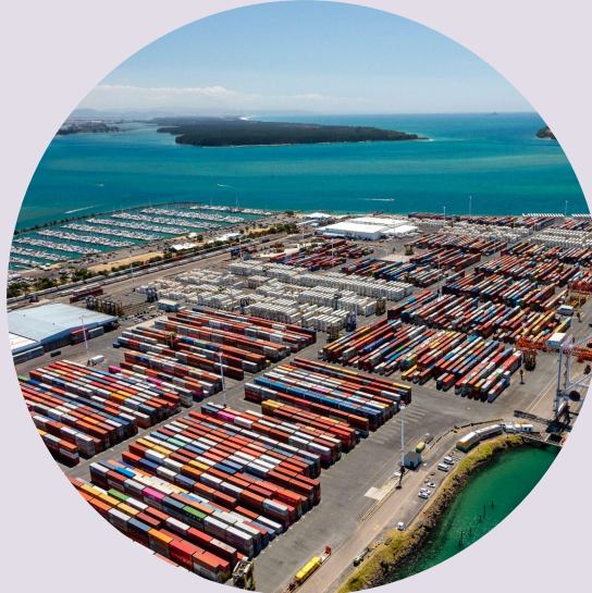
6 Kalmar hybrid straddle carriers and 1 electric straddle carrier to Port of Tauranga, New Zealand
